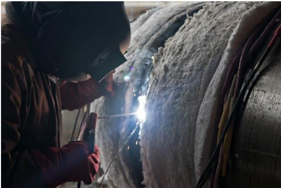
Figure 2.16. Welding with Preheat (Ueda and et al., 2012)
