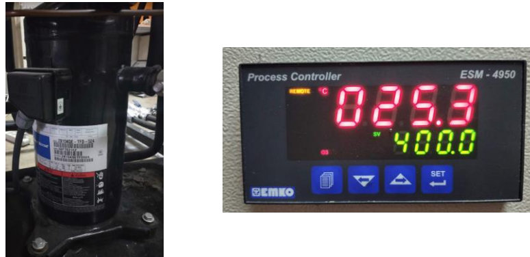
Figure 3.8. The scroll compressor in the system (left) and the on/off relay-based process controller (right)
